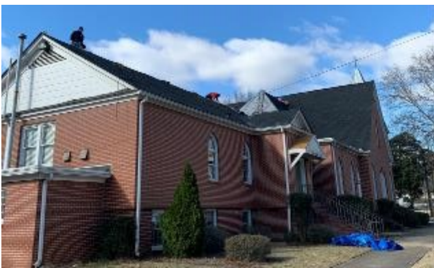
We got a new roof this month!
